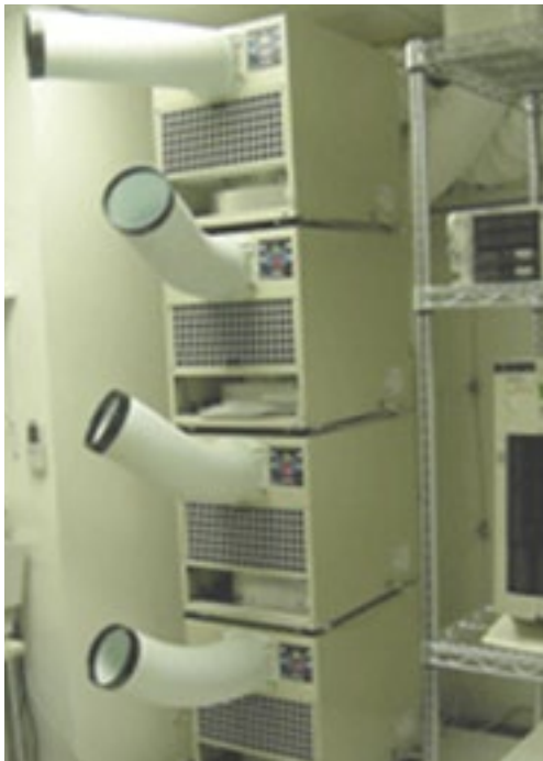
Figure 4. For Tight Spaces, the CoolCube 10 Portable Units can be Stacked to Provide Spot Cooling to Multiple Hot Spots [5]
